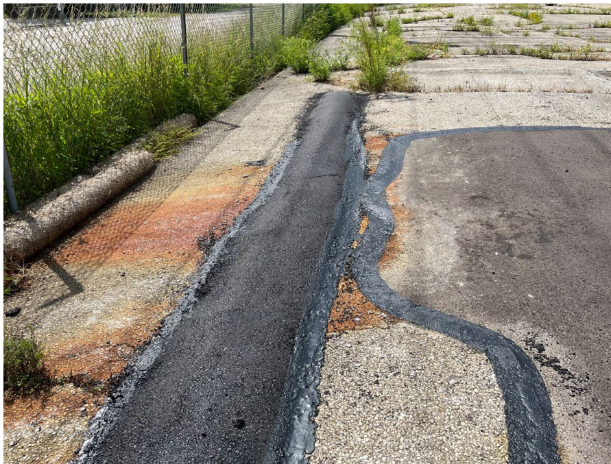
Photograph 1 – New 6-inch curb installed adjacent to east side of infiltration gallery
