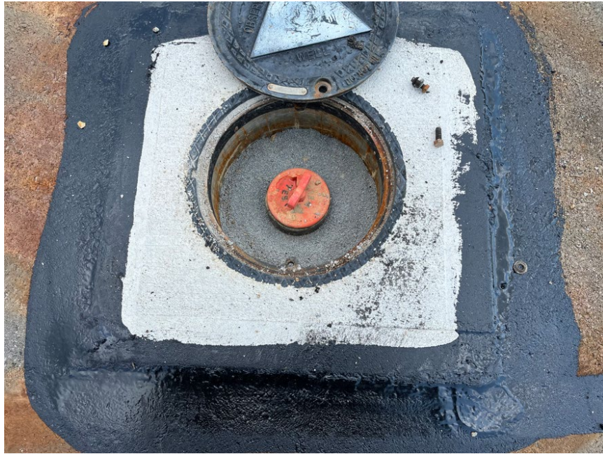
Photograph 5 – Infiltration gallery injection point with bentonite seal.
