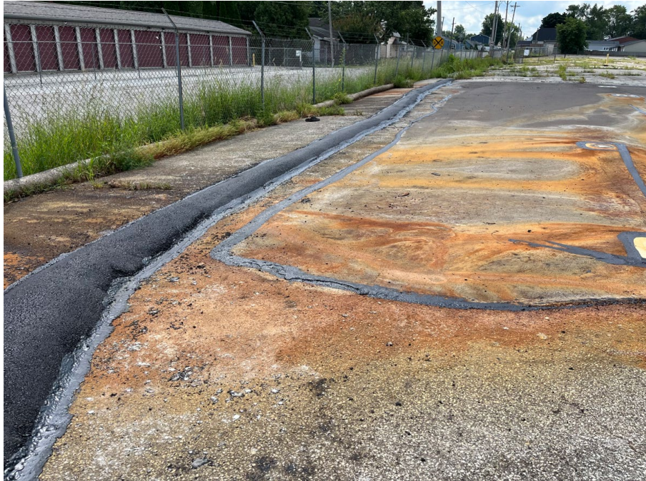
Photograph 1 – New 6-inch curb installed adjacent to east side of infiltration gallery
